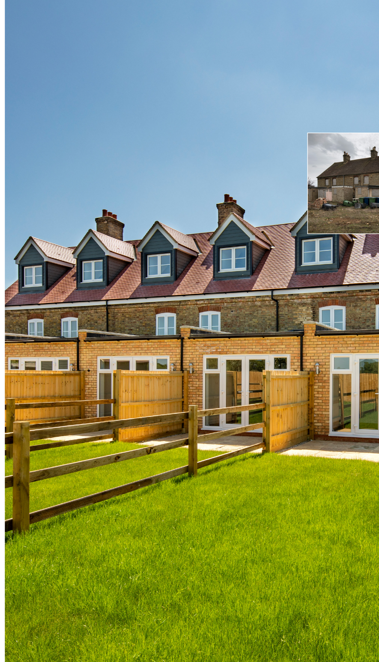
Early 20th century former farm workers cottages located on the edge of Gamlingay village, Bedfordshire are now fully refurbished and extended to provide modern open plan living downstairs and a master suite on the top floor.
